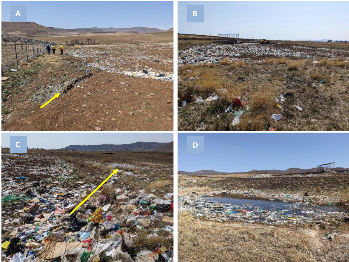
Figure 21: The Barkly East Landfill Site. A) Stormwater diversion berms have been compromised in certain areas. B) The placement of waste within the cells has not been coordinated. C) A trench has been dug through the cell wall to drain the cell to the leachate pond. D) The leachate pond has been choked with waste.
