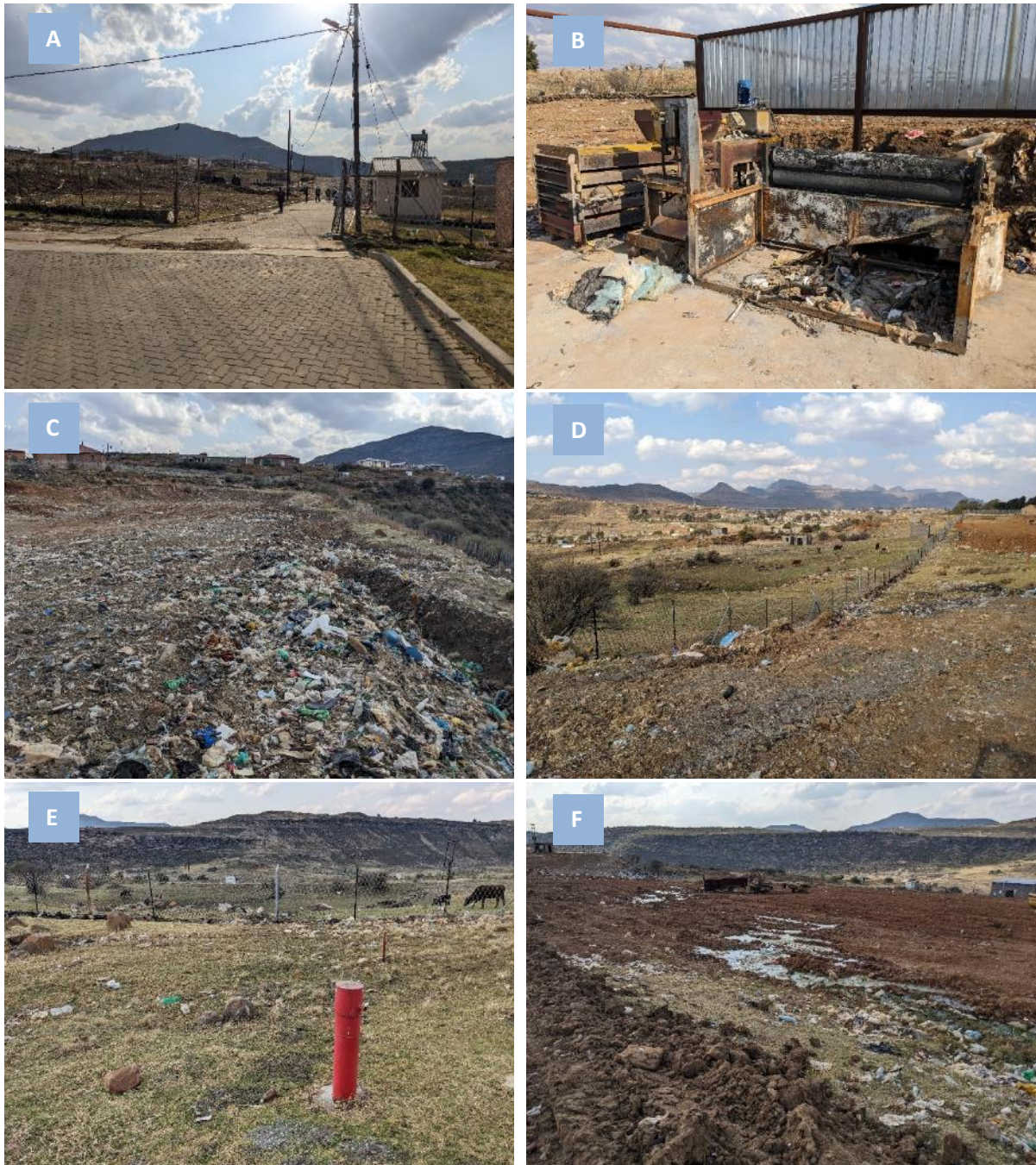
Figure 16: The Sterkspruit Landfill Site. A) Entrance with gate house on the right, B) Part of the recycling facility that was burned down. C) Waste body which has been partially covered with cover material. Note the close proximity to houses along the site boundary. D) Run-off from the site drains off-site to a small wetland area. E) One of the two monitoring boreholes on the site. F) The potable water line to the gate house was leaking, resulting in a flow across the site.
